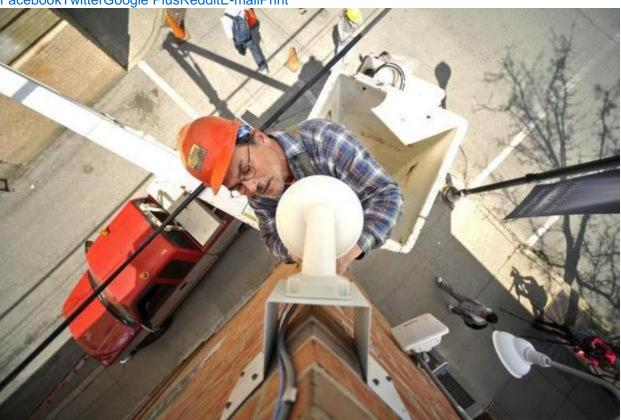
Electrician Scott Koenig installs a security camera on a building at the Allen St. and Calder Way intersection. State College is in the process of installing 71 cameras in the borough. NABIL K. MARK — CDT photo |Buy Photo
